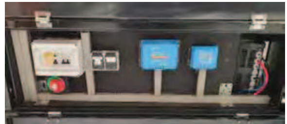
Figure 23: New DC installation in the Tuktuk
