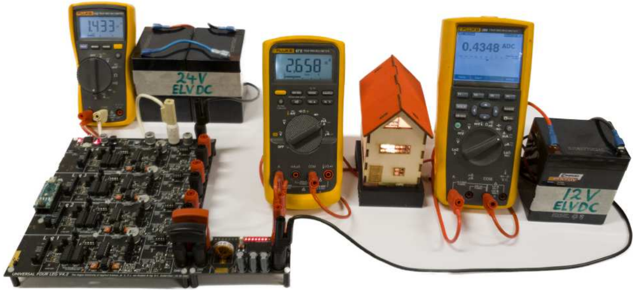
Fig. 8. Experimental setup used to test an active DC-grid system. From left to right: the U4L with a 24V DC-link battery and current measurement, a current controller PCB with current measurement, a resistor load and fixed 12V DC voltage battery with current measurement.
